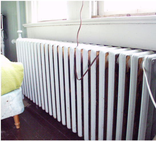
Figure 35 View of radiator in Room 203, which was typical of those installed in the 1930s. (NPS-SERO-CR, 2002)
